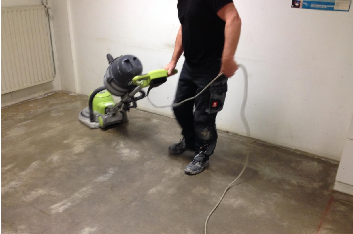
Sanding of primer with a sanding machine
